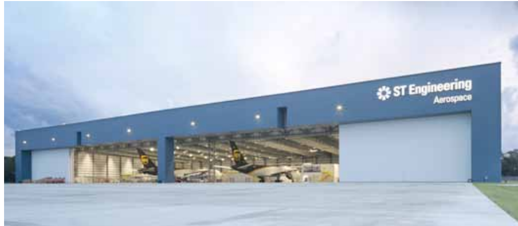
The new airframe MRO facility in Pensacola, Florida, U.S..
