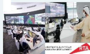
Dubai iTraffic Road Command & Control Centre with state-of-art technologies
